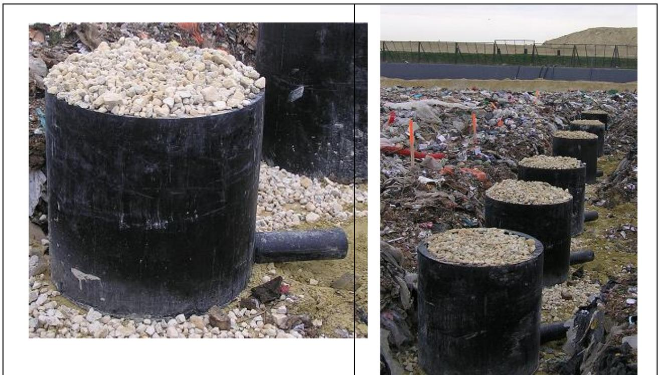
Picture 2 : Lysimeters set up in the landfill cell
